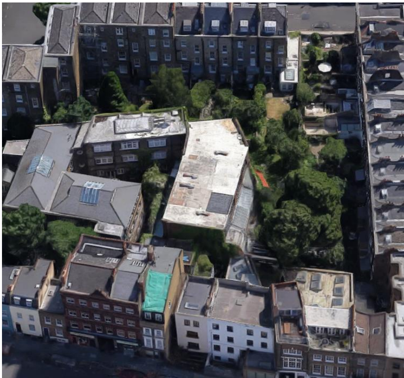
Aerial view of the site in an easterly direction
