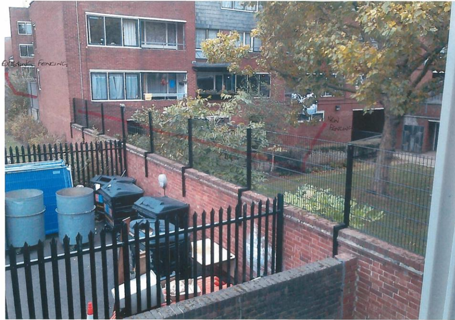
North-eastern boundary wall backing onto gardens to Chalbury Walk showing new fence was installed
