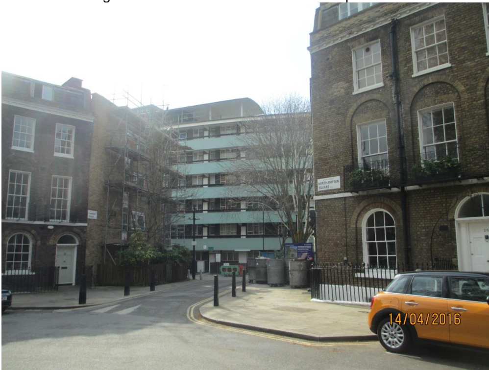
Image 4: View of front elevation from Northampton Square
