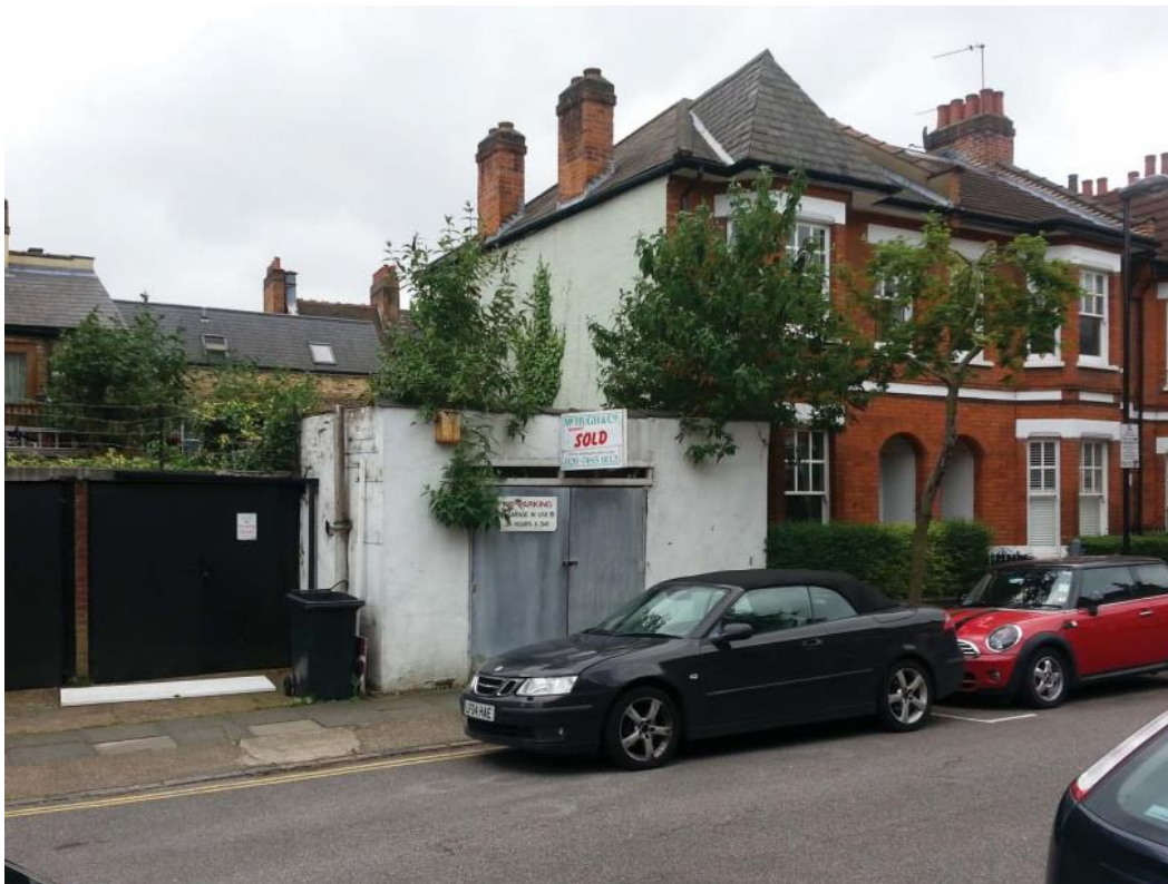
Existing Street view of Application Site
